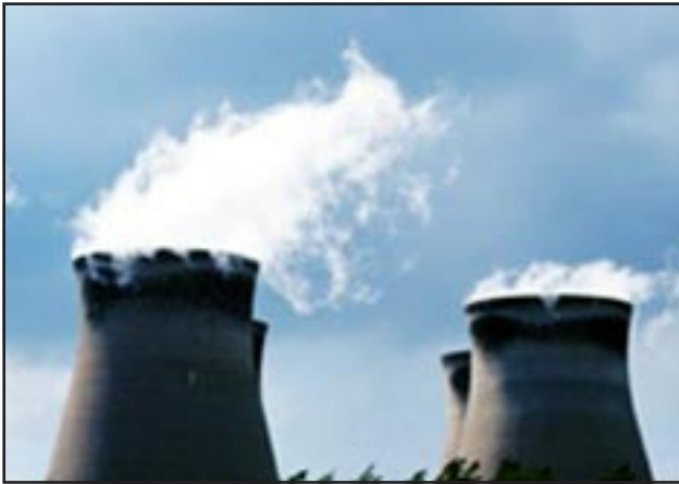
Hrazdan power plant
