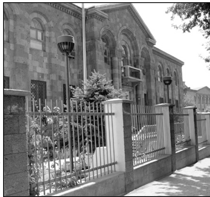
The newly acquired AMAA Headquarters in Yerevan
