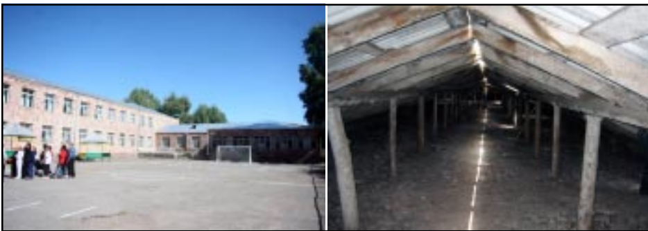
Gavar special school roof after restoration and before
