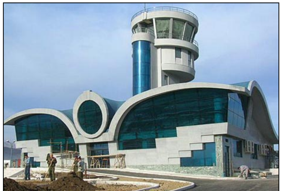
Stepanakert airport terminal under construction
