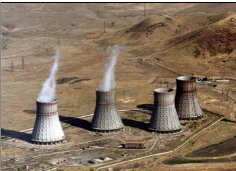
Metsamor nuclear power station
