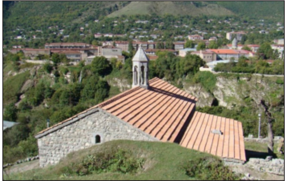
Renovated Sourp Astvatzatzin Church near Goris
