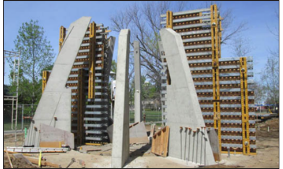
The monument under construction
