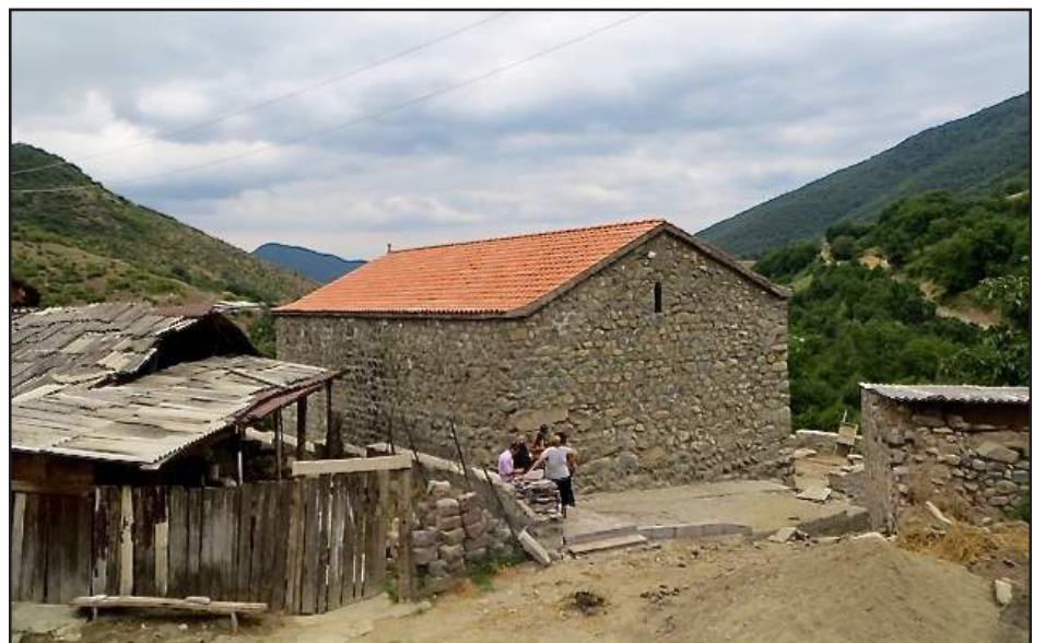
Shikahogh village Sourp Stepanos Nakhavegah church before and after restoration
